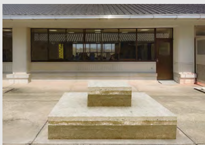
Image of the Rammed Earth Project in Seto "Convex"
