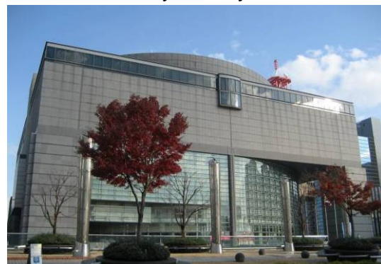
Aichi Arts Center, located in Sakae (downtown Nagoya)
